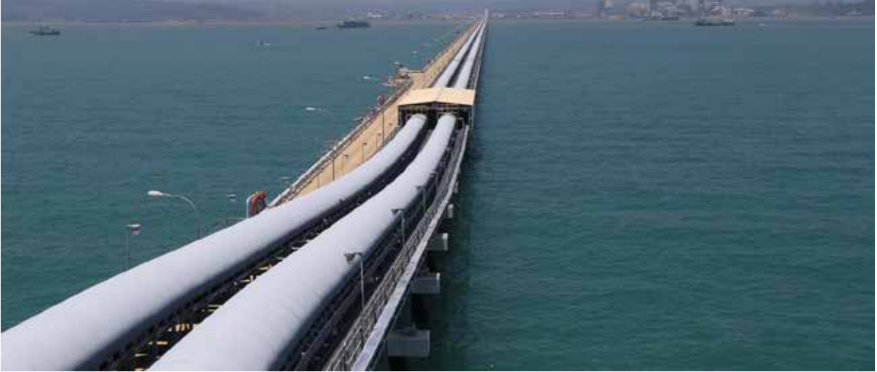
Construction of coal transport jetty
