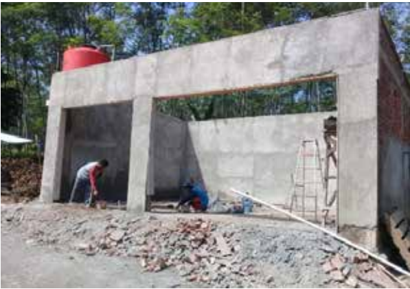
Supporting trash bank storage construction in Ujungnegoro village
