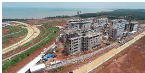
Batang Integrated Industrial Park
