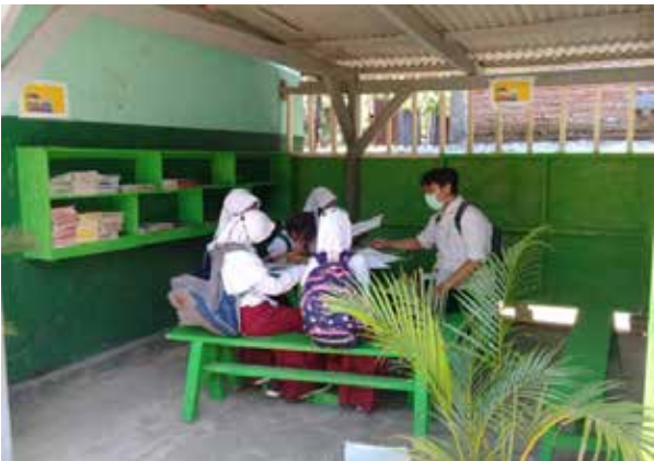
School reading corner renovation in MI Salafiyah, Beji village
