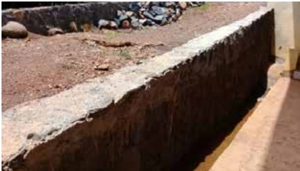
Supporting water sanitation renovation in Darussalam Islamic Kindergarten, in Karanggeneng village
