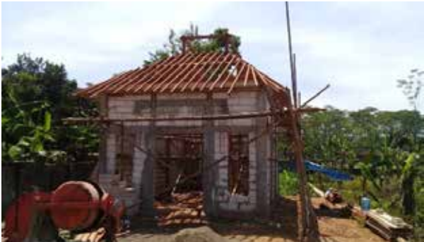
Supporting Mushola Makam mosque renovation in Beji village
