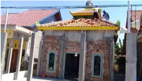
Supporting Al Hikmah Mosque renovation in Ponowareng village
