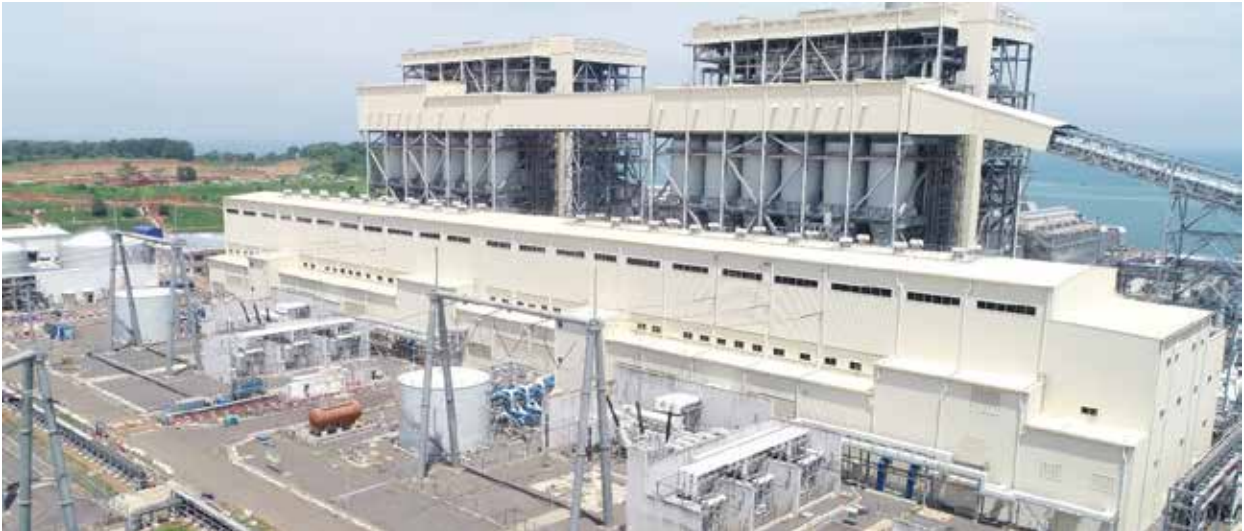
Construction of Turbine and Boiler Unit 1 & 2
