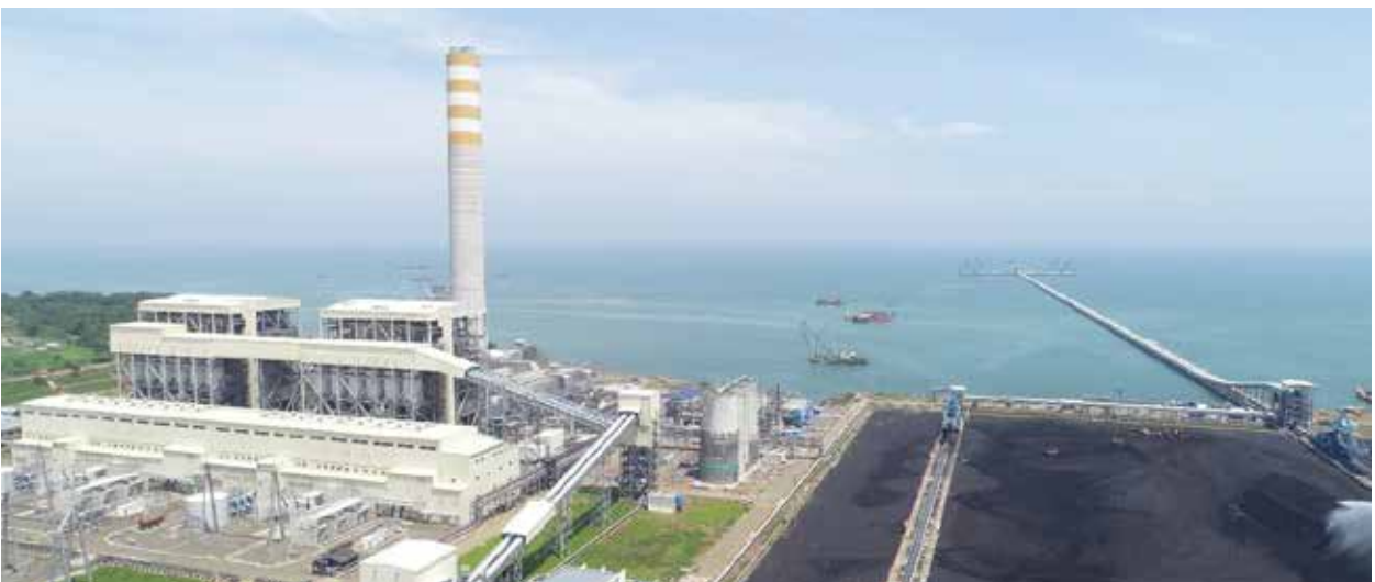
Aerial view of CFPP construction
