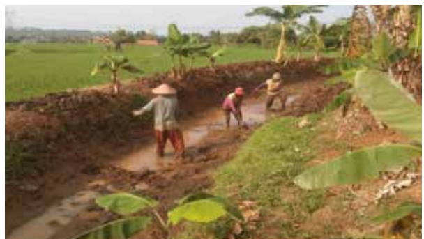
Improvement work of irrigation channel to A & B2 area
